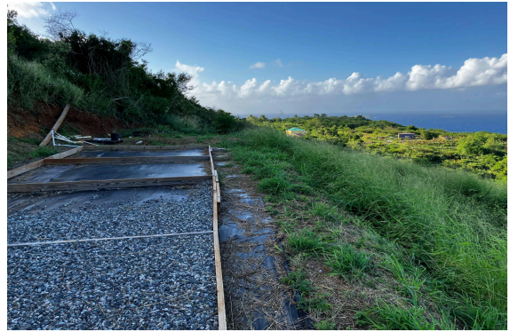
Gravel beds to support an Irrigation Reservoir, a conservation practice cost-shared in an EQIP contract in the Bordeaux region of St. Thomas, USVI. The cost of the practice far exceeded the cost-share but will improve the producer's reliable water supply for fruit tree irrigation.
